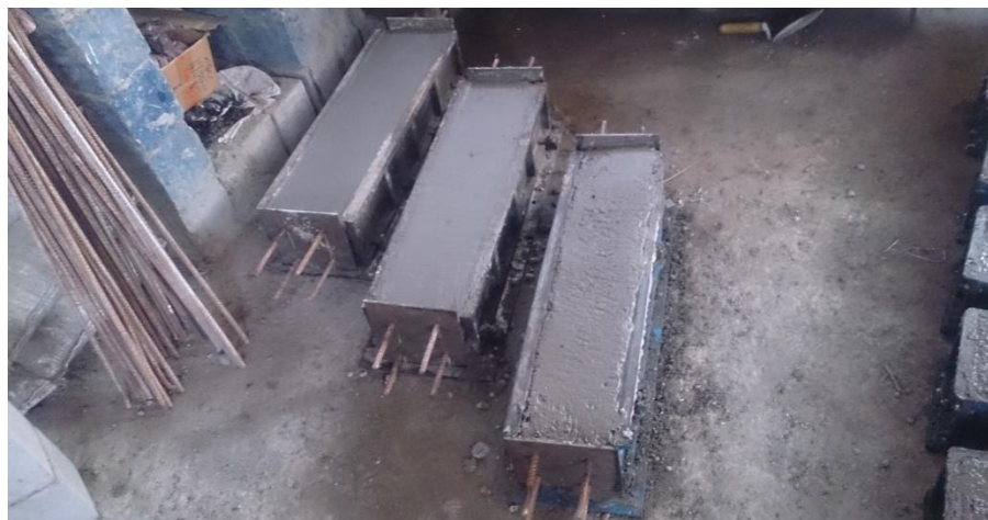
Fig.5 Casted beams specimen with reinforcement
