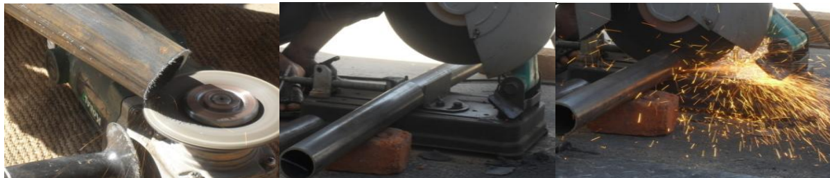
Fig 3:- Cutting & preparation of Specimen to required Length
