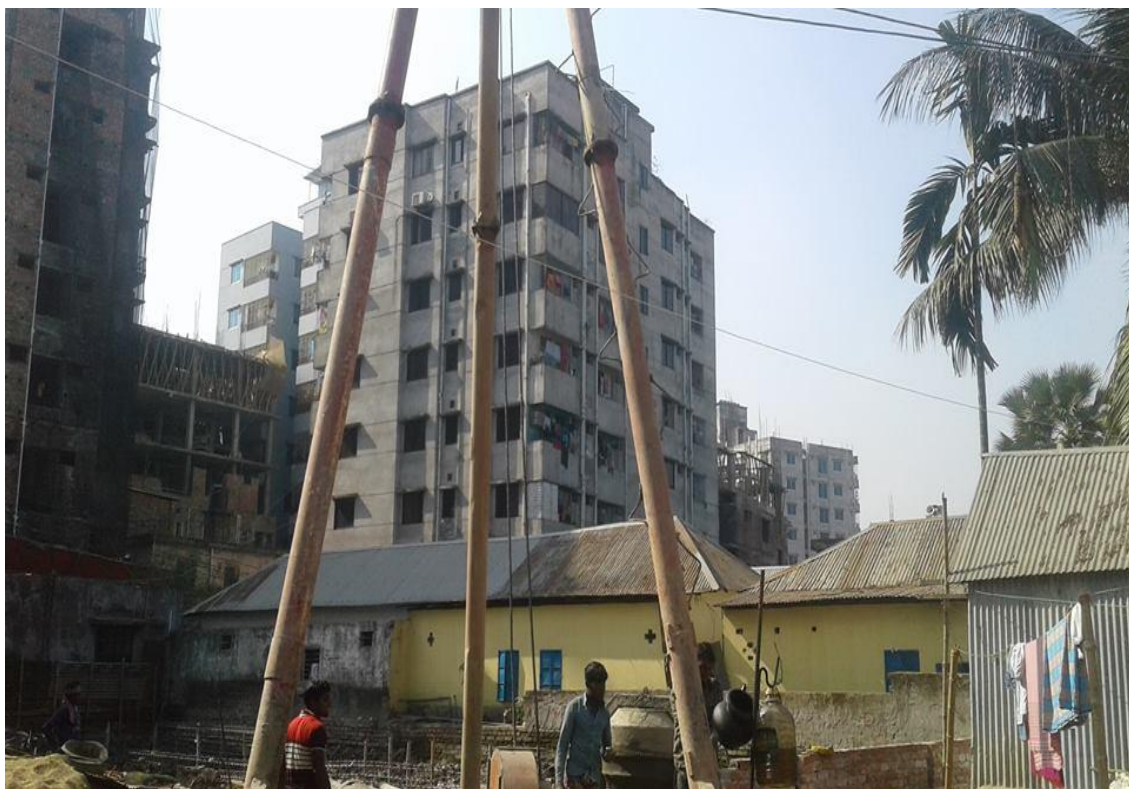
Figure 1: Drive of sand pile
